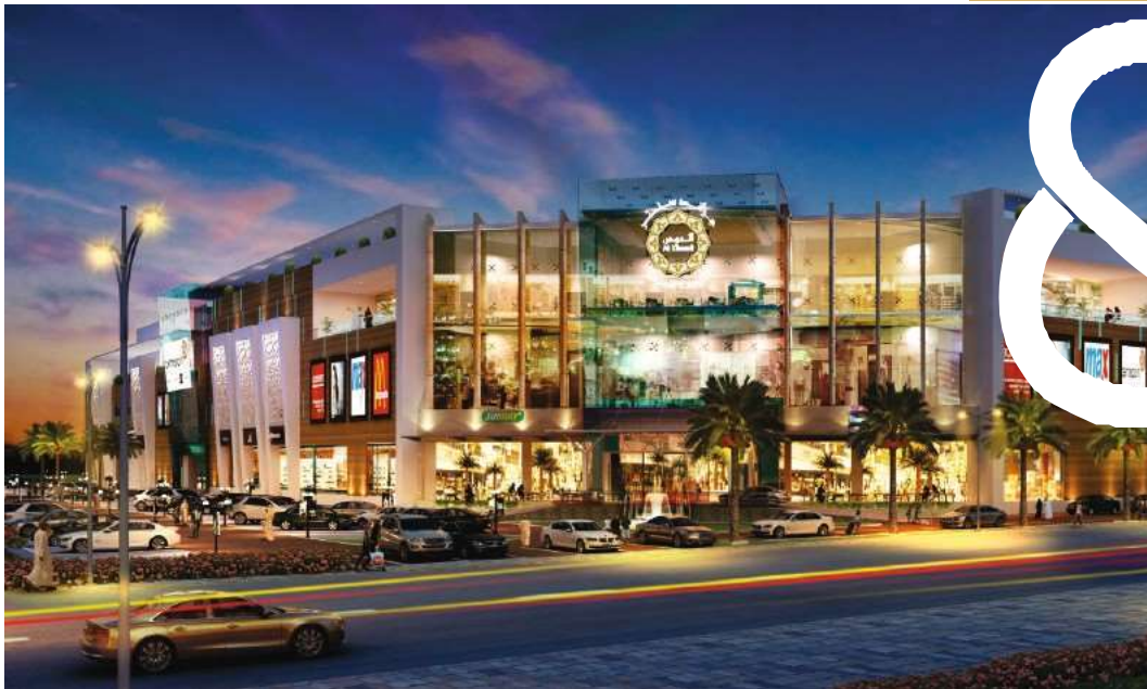
AL KHOUD MALL, Muscat (Area: 100000 sq.Mtr) Scope: HVAC, Electrical, Plumbing & BMS Design Client : EIDC
