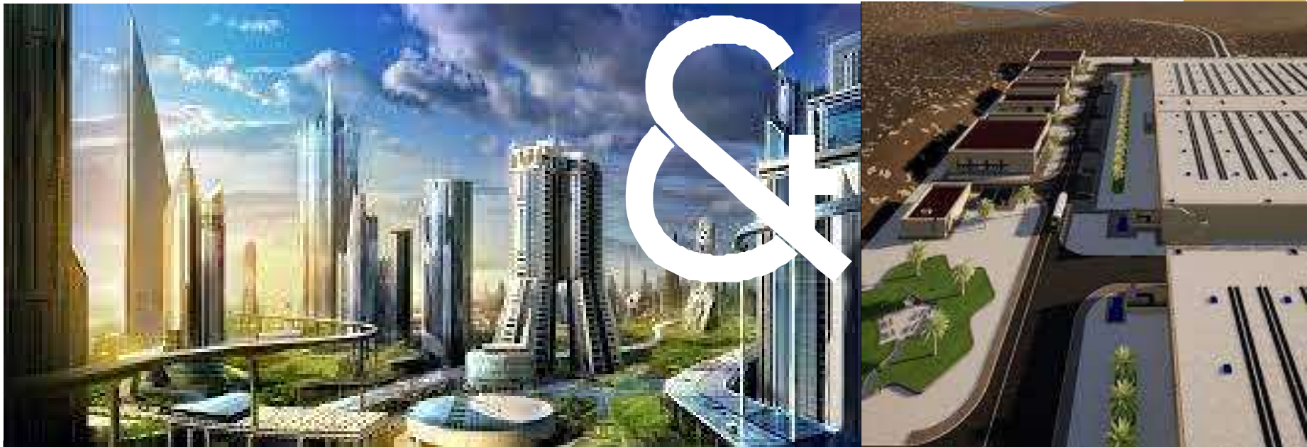
NEOM, NER & WICR Site Utility buildings, Saudi Arabia
